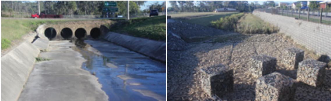
Images of urban drains. Left: Urban drain showing hard surfaces and loss of natural stream attributes. Right: Urban drain designed with rock-filled gabions to reduce flow velocity but note lack of bank-side vegetation and uniform sides, Gladstone.
