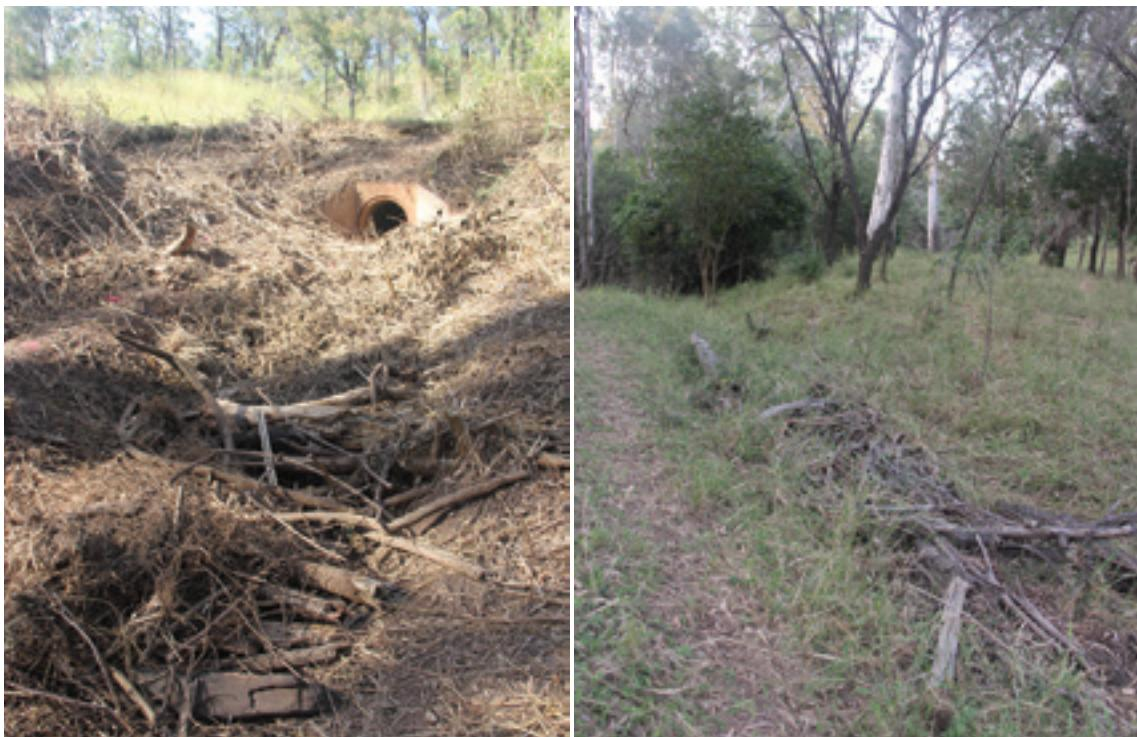
Images of using woody debris. Left: Using woody debris to reduce flow velocity, Boat Creek, Yarwun. Right: Woody debris used to minimise gully scouring Double Creek, Calliope.
