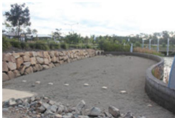
Image of sedimentation pond at Riverston Rise Estate, Boyne Island. Stormwater enters via the drain, spreads and slows dumping of its sediment load. The concrete ramp allows access for maintenance.
