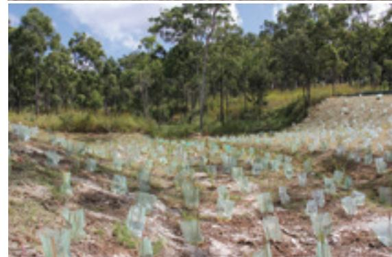
Images of stabilisation using plants and seeds. Top: Seeding a fast growing cover crop, in this case a grass, to help stabilise a bare earth bank. Note the surface has been ripped along the contour. Bottom: This creek crossing site has been battered, geofabric has been installed, the site seeded and then planted with a range of native tubestock. (Images courtesy of CVA Gladstone.)
