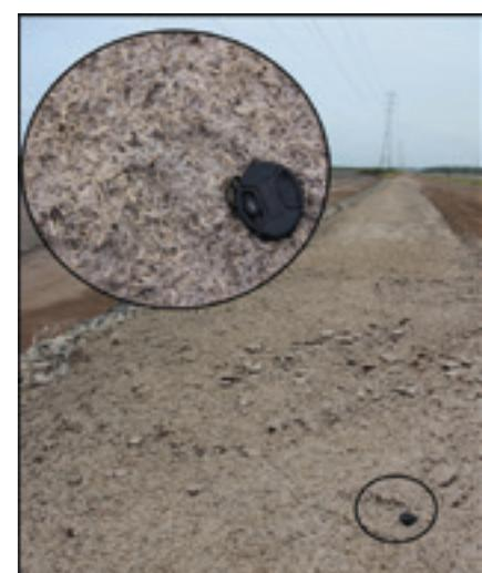
Image of hydromulching; camera lens cap included as a size reference.
