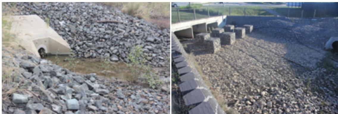
Images of rock reinforcement in drains. Left: A stormwater drain outflow with rock armoured sidewalls, Gladstone. Right: An urban waterway using rock-filled gabions to break flow and reduce velocity, and rock-filled mattresses to prevent scouring of the bed, Gladstone.
