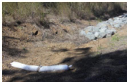
Images of socks. Far left: Hay bales installed to minimise contaminants entering a wetland from an industrial site, Wapentake Wetlands, Gladstone (Image courtesy Conservation Volunteers Australia, Gladstone). Left and above: Geofabric sandbags and silt fence to minimise sediments in run-off into creek systems, Boyne Valley.
