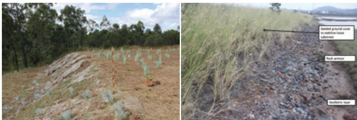
Images of slope battering. Left: A battered slope leading into a creek crossing the Western Basin haul road, Gladstone (Image courtesy of CVA Gladstone). Right: A battered slope showing an integrated approach to erosion control: directly seeded, geofabric base layer and rock armour, Gladstone.
