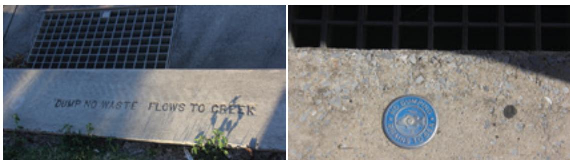
Images of commercially available drain components and plaques labelled with messages to protect waterways, Gladstone.
